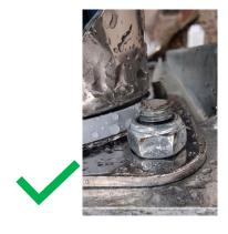
If the locknuts are correctly installed the trolley base is safe to use and you may use it as normal.
